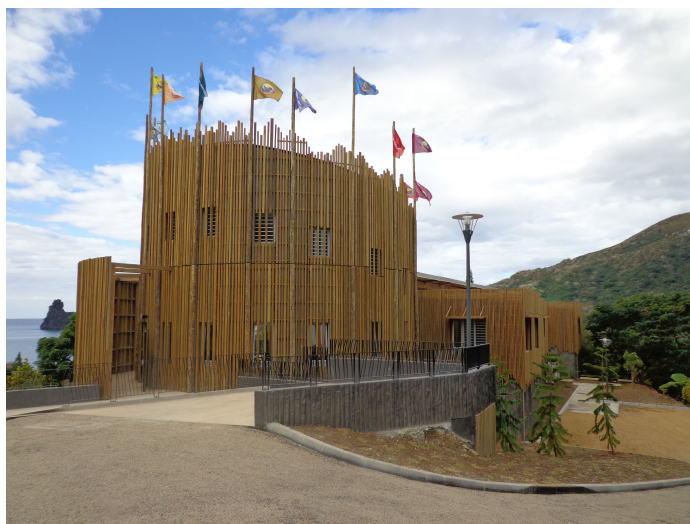
Mesh cladding on Hienghène city hall – By: Les Charpentiers du Nord - New Caledonia © Henry Séchet, Scierie de Netchaot
